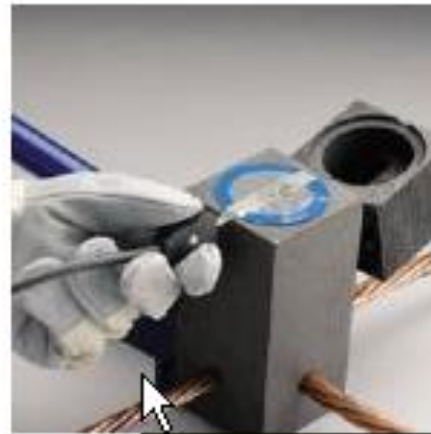
CADWELD PLUS installation - s
